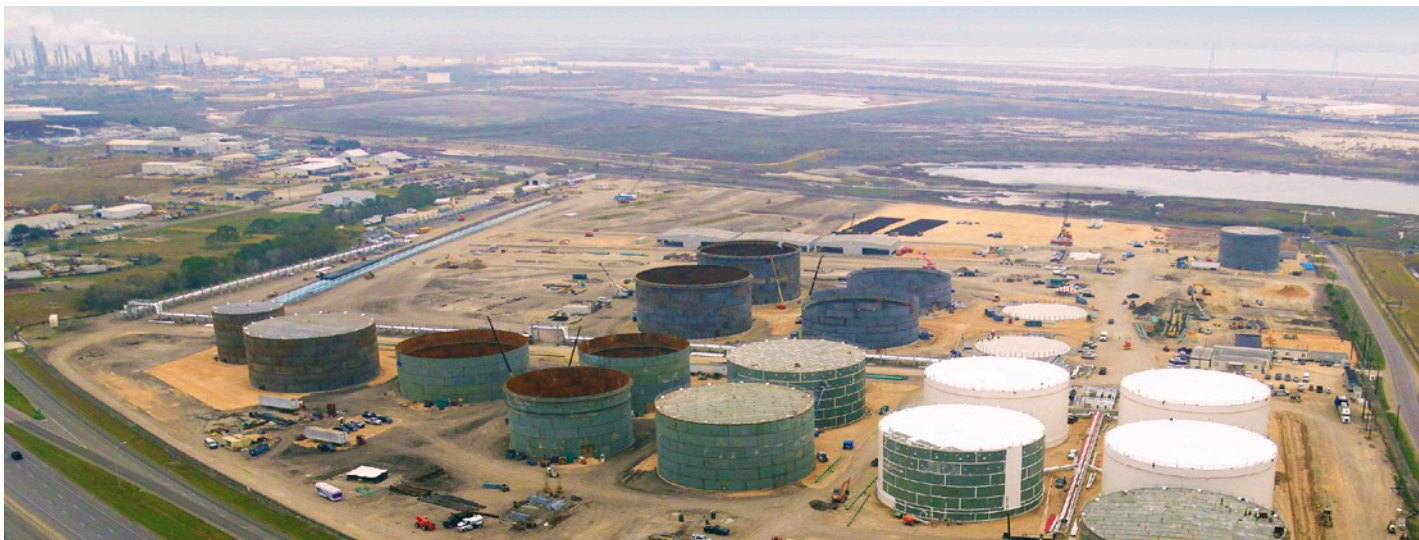
Oil storage facility under construction, Corpus Christi, Texas.
