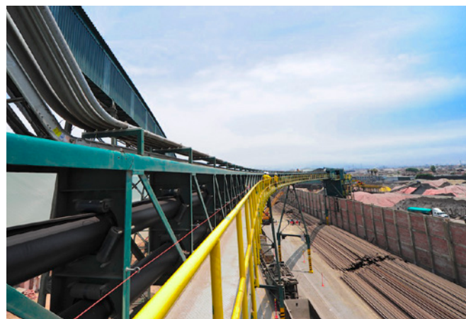
Newly constructed conveyor, Port of Callao, Peru.
